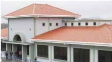
Western Regional University Center - CUROC
